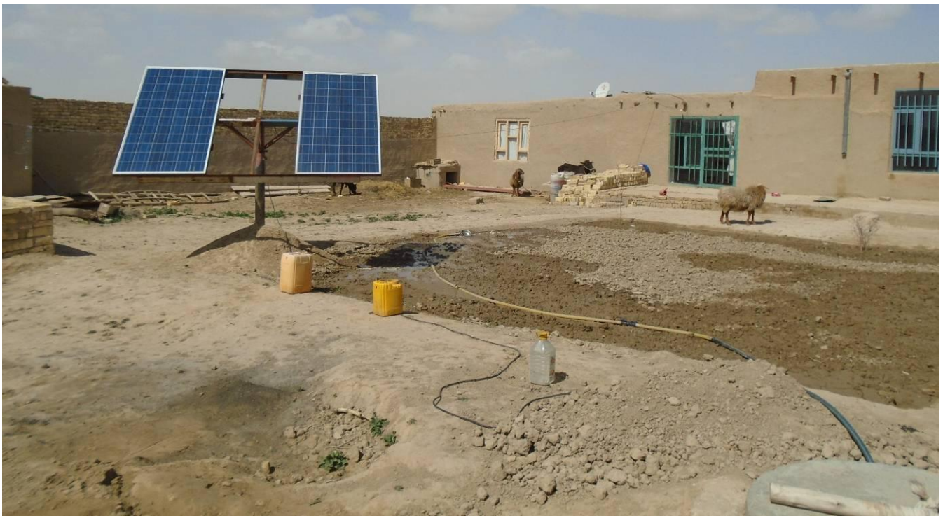
Investing the returns of her dairy business and the sale of two calves, each at AFN 18,000 and AFN 23,000, respectively, Sughra made a borehole and installed a solar water-pump system to access clean water.
